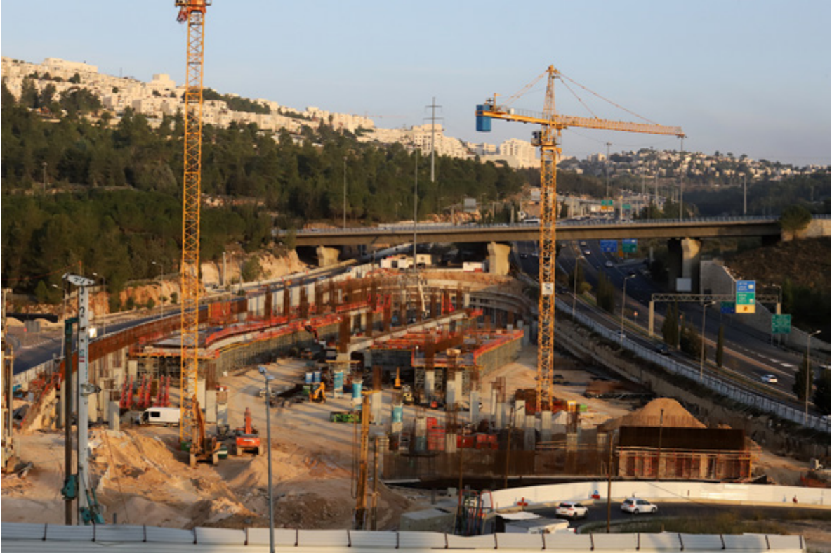
The "park and ride" lot under construction in the settlement of Ramot
